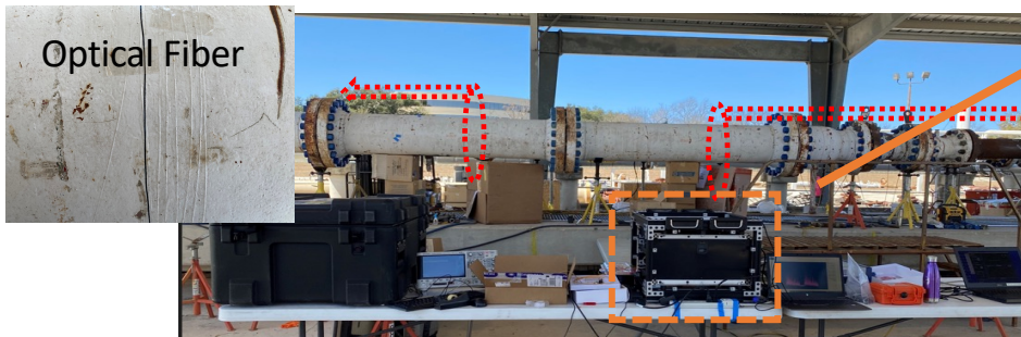
Operating NG Pipeline
